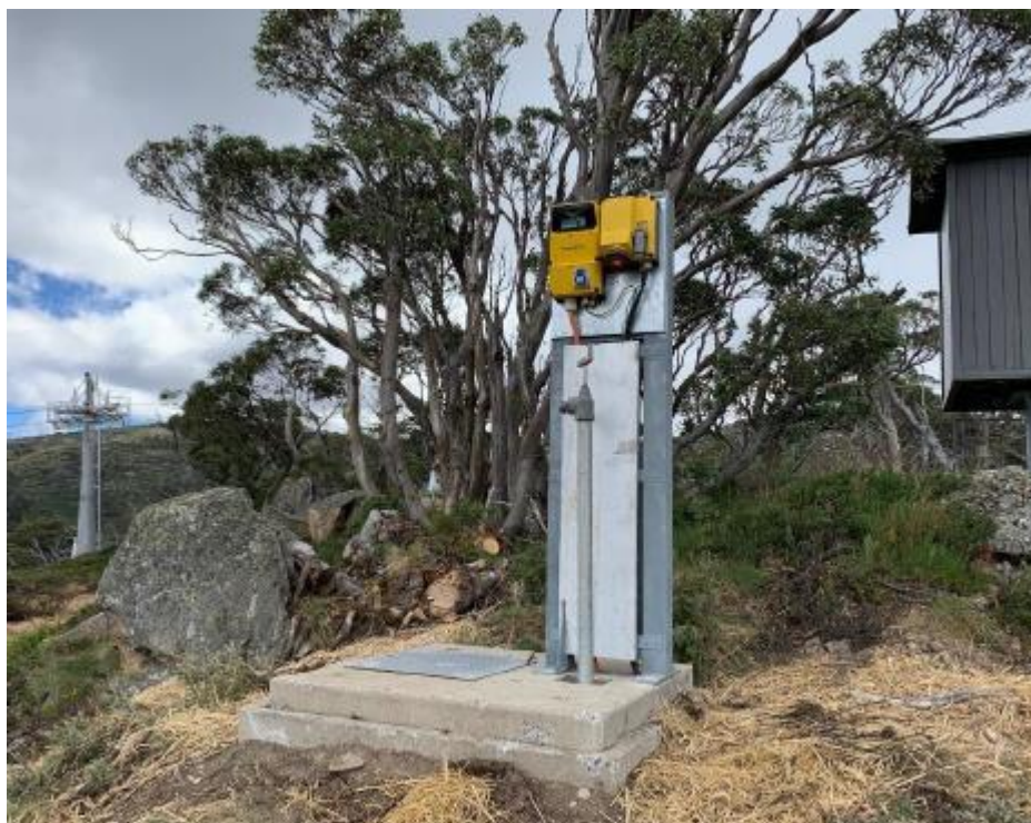
Figure 4 | Example of prefabricated concrete pit, with hydrant and power outlet (Source: Applicant's documentation)
