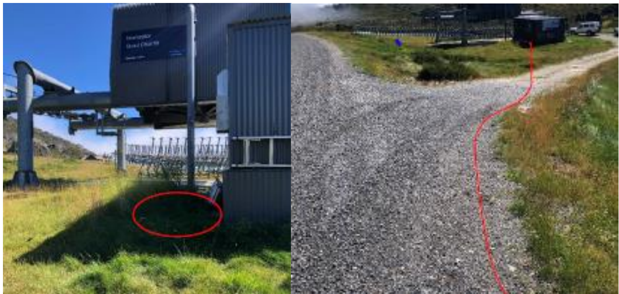
Figure 2 | Site 1, adjacent to Interceptor Quad Chair bottom station, and trenching (red line) up through existing access track and Perisher Creek Road to Site 2, approximately 70 metres along the road edge (Source: Applicant's documentation)
